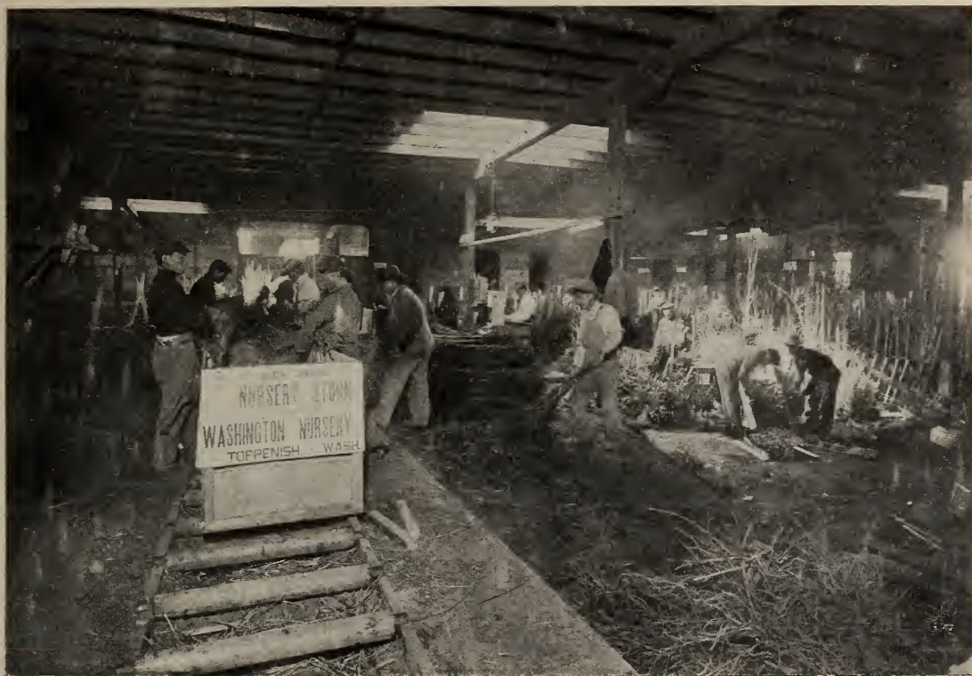
PORTION OF PACKING HOUSE.
